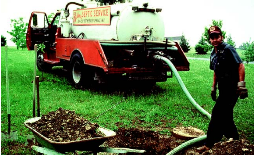
Septic tanks should be pumped out every three to five years to prolong the life of the system.
