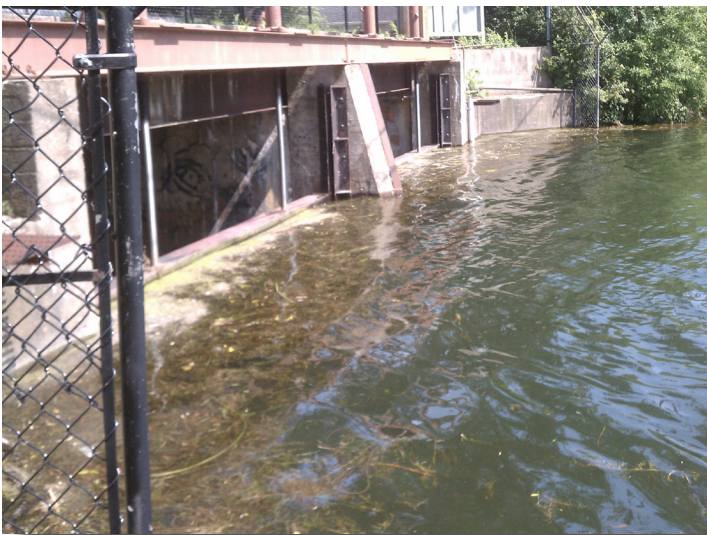
Outlet gates in the closed position
