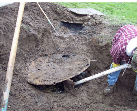
Digging up a failed onsite wastewater system.
