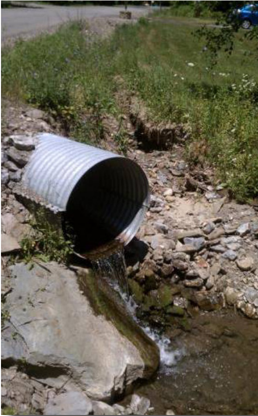
Culvert that is undersized and difficult for fish passage-needs to be embedded.
