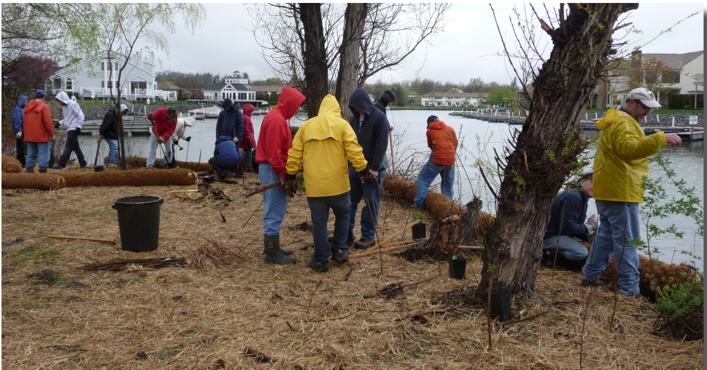
Atwater Meadows shoreline stabilization project. Project completed with the Canandaigua Tennis team installing the plantings and coir rolls to stabilize the shoreline.
