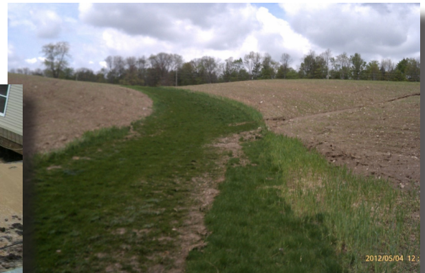
Grassed waterway was installed to prevent erosion and filter runoff (above).
