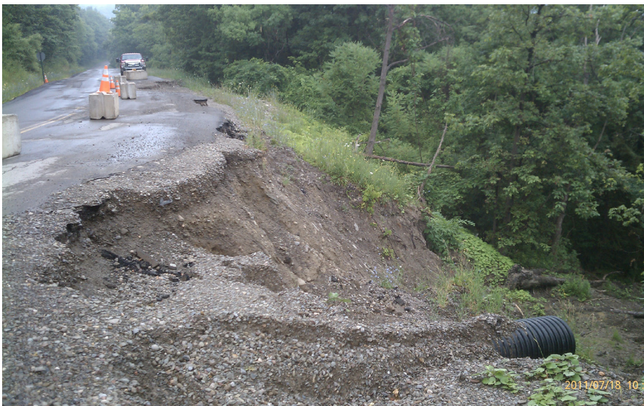
Major storm caused the water to overtop Dug Road in Naples and cause major damage and tremendous costs. A proper culvert was installed to handle the flow and debris load.
