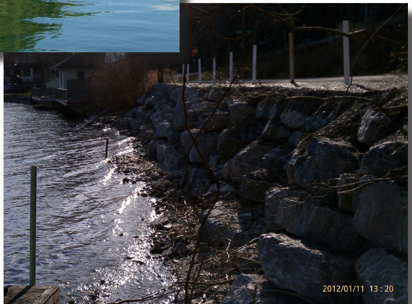
Rock stabilization along an existing road was the only solution after the floods of 2011.
