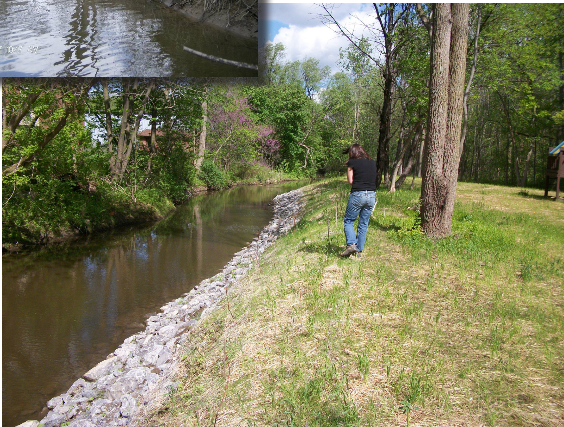
Project along Sucker Brook - project completed with the Town of Canandaigua installing toe stone protection and plantings on the upper two thirds of the bank.
