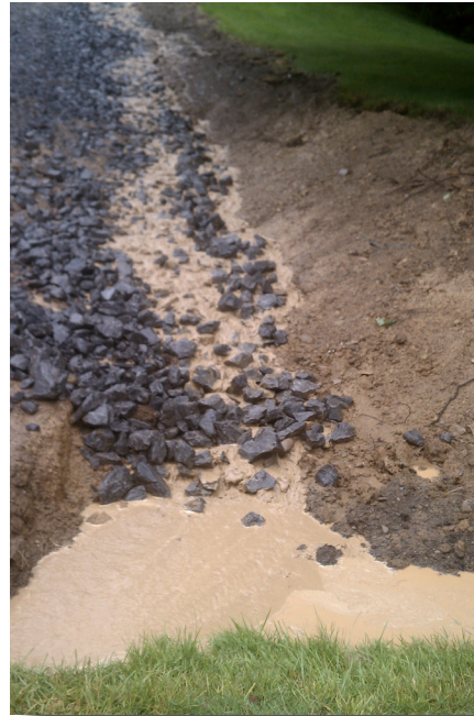
Inadequate erosion and sediment control measures on the uphill portion of this steep slope development caused significant sediment to leave the site.
