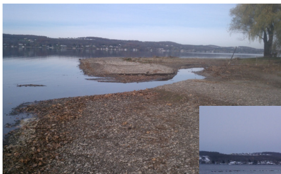
Deep Run before dredging with significant sediment deposits at the outlet (left).
